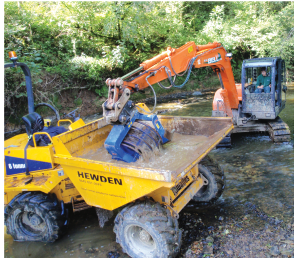
Gravel cleaning at Luffincott
