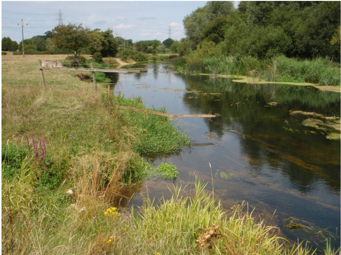
Photo 6. Upstream deflector and fry refuge area completed
