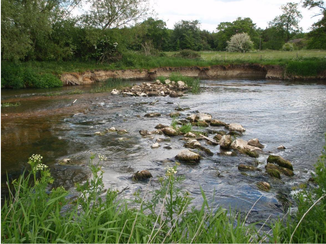
Photo 2. Glens Weir after re-profiling and bank stabilisation
