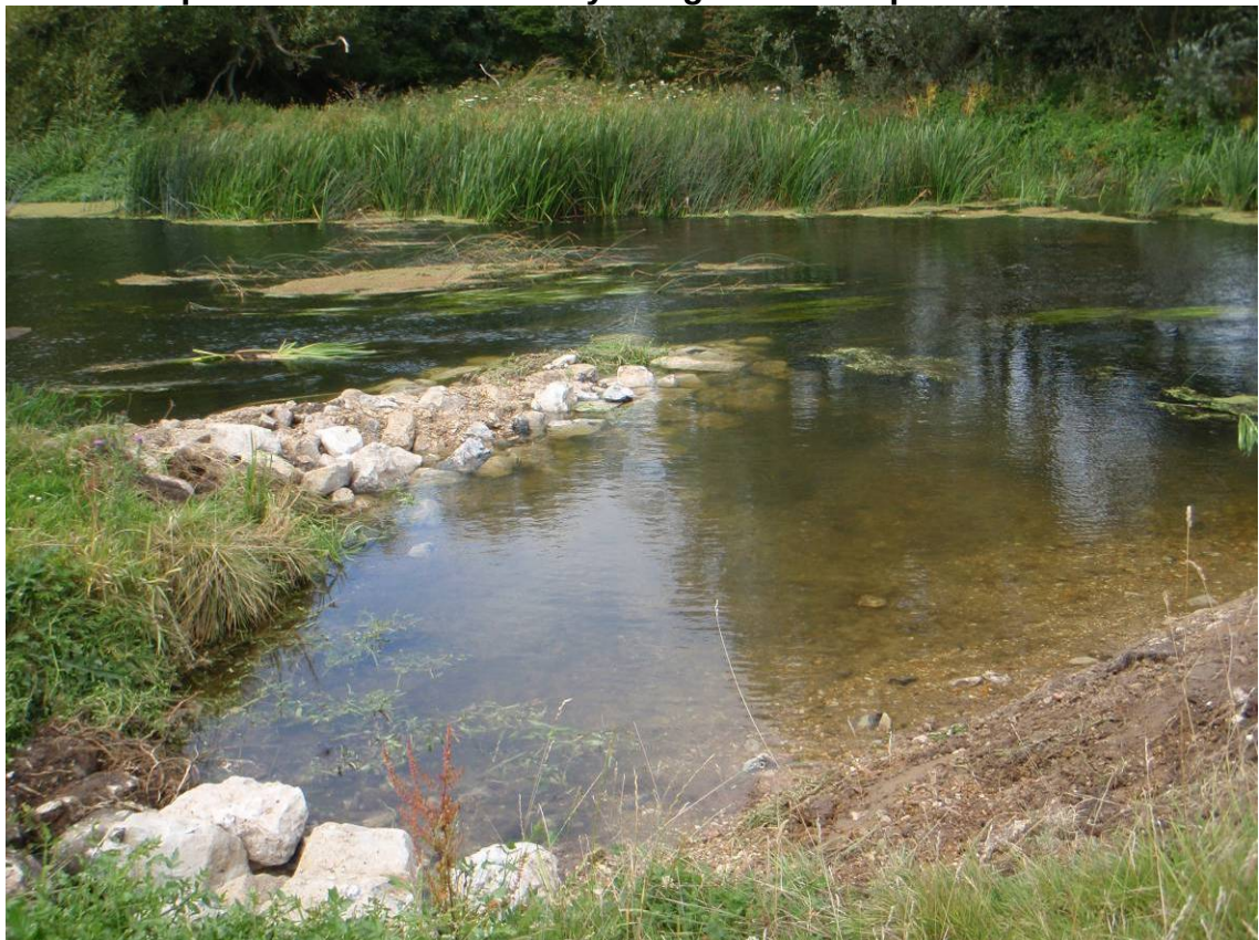
Photo 6. Upstream deflector and fry refuge area completed
