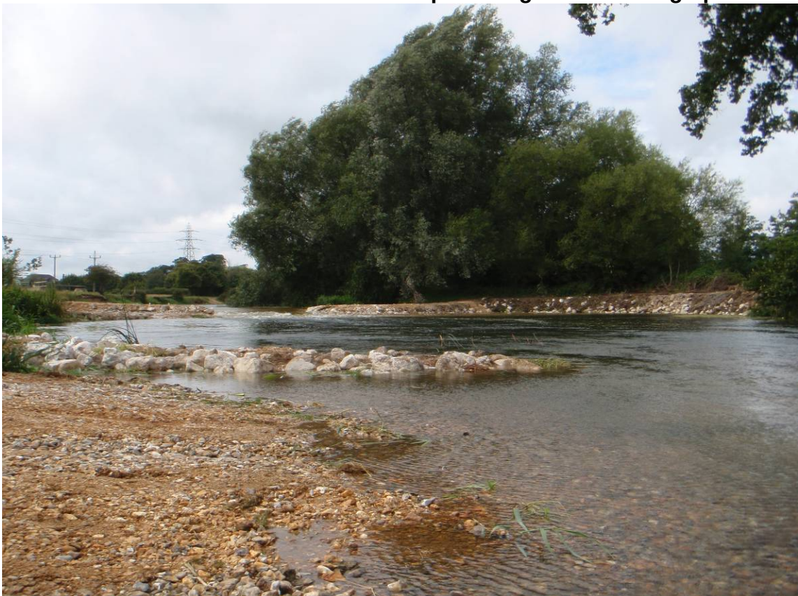
Photo 10. Downstream deflector and re-profiled gravels looking upstream
