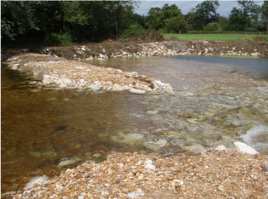
Photo 2. Glens Weir after re-profiling and bank stabilisation
