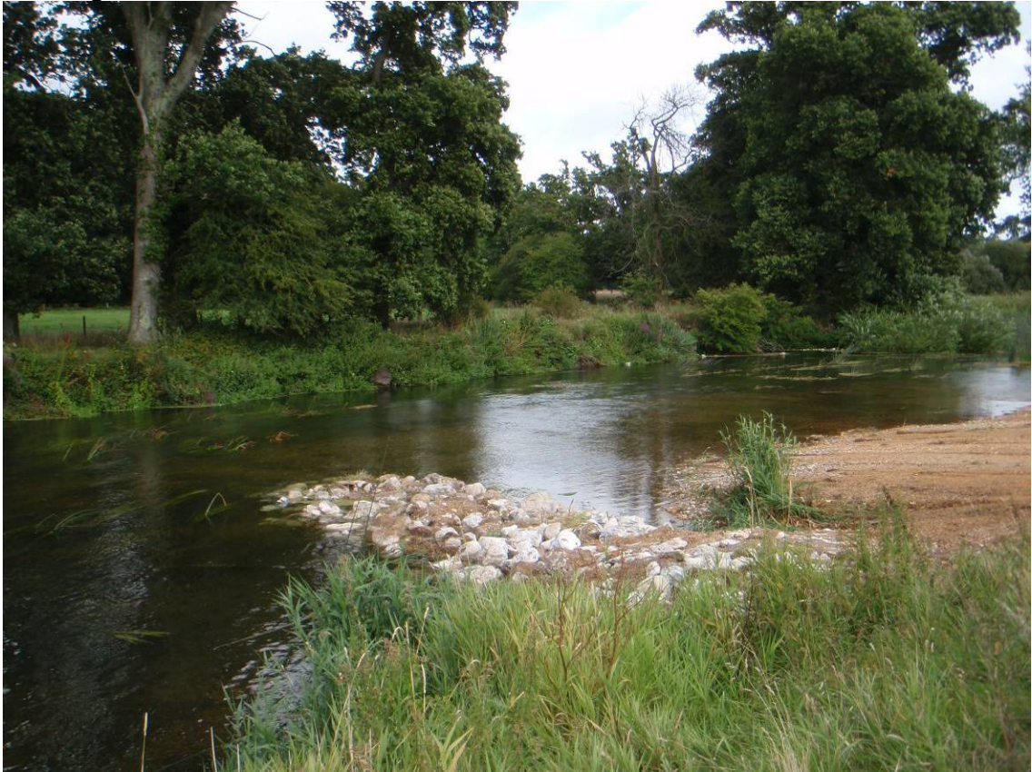
Photo 10. Downstream deflector and re-profiled gravels looking upstream
