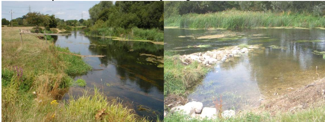
Downstream deflector and re-profiled gravels
