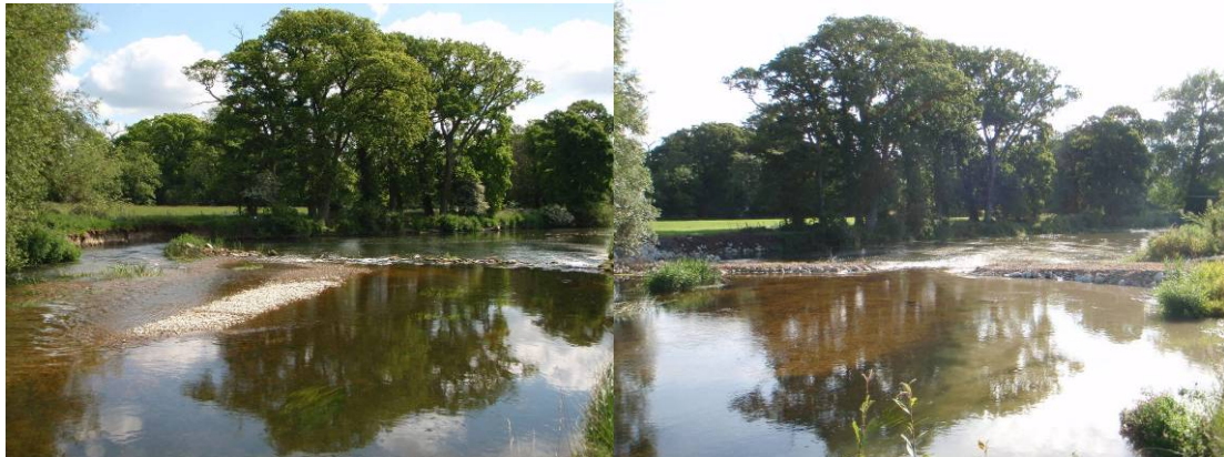
Upstream deflector and fry refuge area before and after
