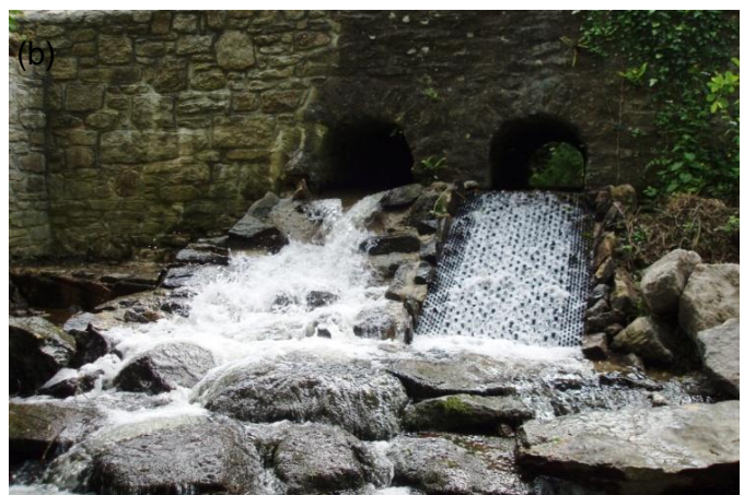
The undermined bridge at Retyn on the River Gannel (a) and the newly installed rock ramp and eel pass (b)
