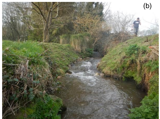
Removal of a culvert (a) on the Polgooth stream with bank re-grading and re-turfing (b)
