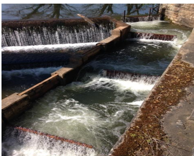
French weir fish pass before (top) and after (bottom) repair
