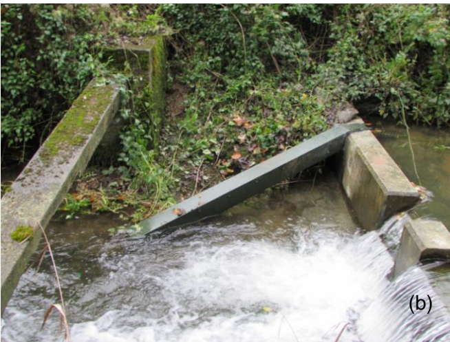
Inspecting the weir (a) before the eel pass and a section of the eel pass (b) on one of the pre-barrages
