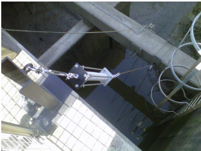
A retarder on a tide flap that slows the closure rate
