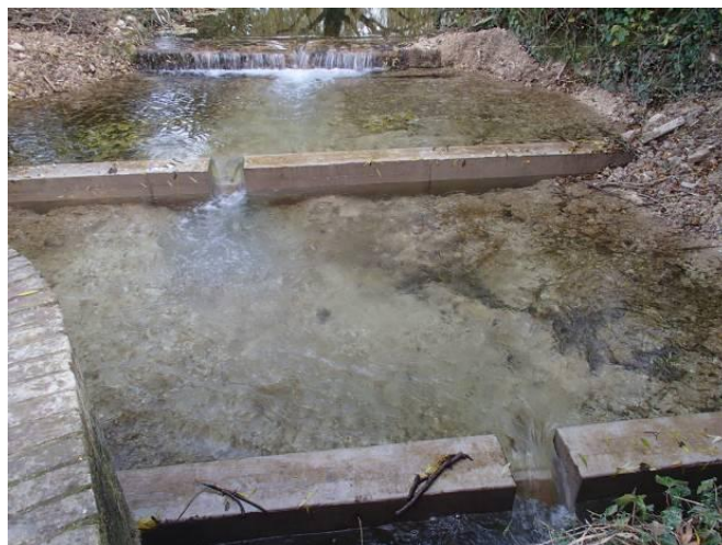
New pre-barrages at Manor Farm Weir, River Tarrant to help improve fish passage
