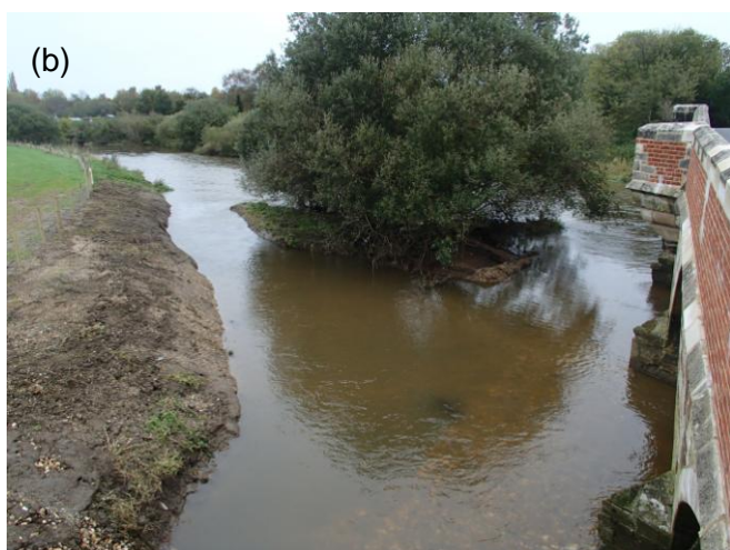
Pre (a) and post (b) work at Julian's Bridge, showing one of the two new high flow channels and fry bay
