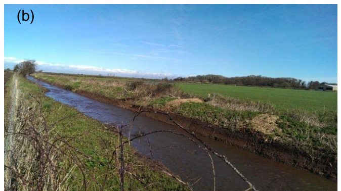
The River Avill before (a) and after (b) de-silting with further improvements planned
