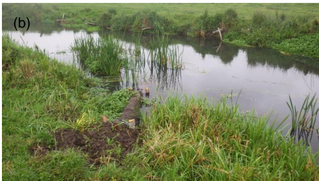
Re-instatement of a gravel beach (a) and LWD to trap sediment (b) on the River Piddle
